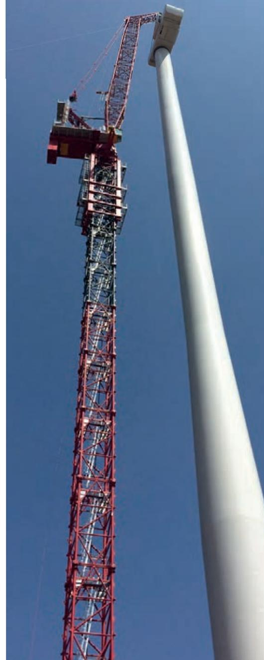
Since turbulent wind can cause resonance and fatigue failure in tower cranes, it must be kept under watch. Here ALE is using a tower crane to erect a wind turbine in Thailand (see the *wind turbine erection* feature on p25 for more info)
